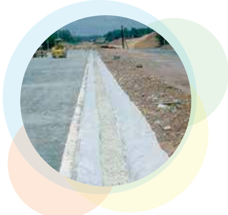
Standard Geotextiles used in a French Drain application.
