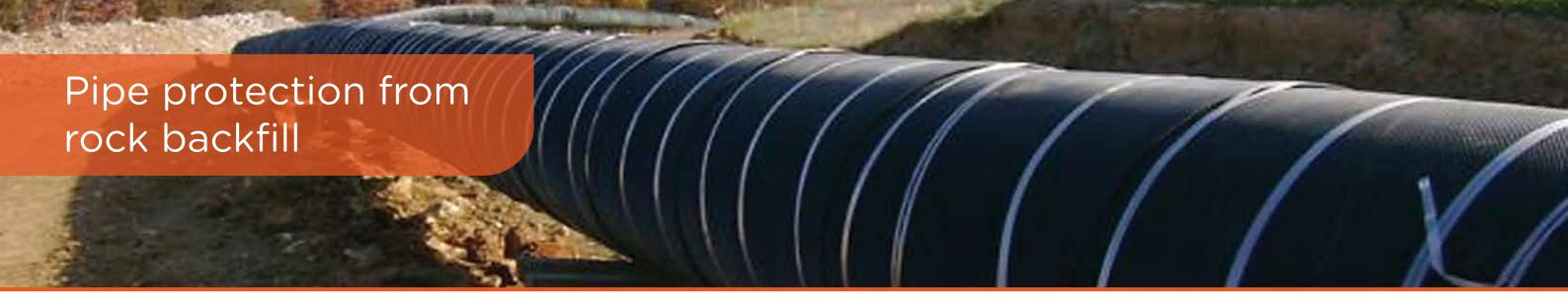
Flexible mesh products are used in major pipeline projects to replace the thick sand collar that would traditionally have been placed to cushion the protective coating around a steel pipe.
