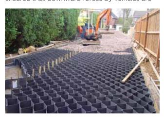
spread laterally reducing loads on the underlying soils. Without the cellular system, the surface would have become compacted and rutted with the forces pushing downwards damaging the tree roots and possibly killing the trees. Geocell was installed onto the level surface on top of a geotextile. The cells were filled with a type 1 road stone and compacted flat. A geotextile and binding layer were installed on top of the cells and the surface finished with small angular gravel.
