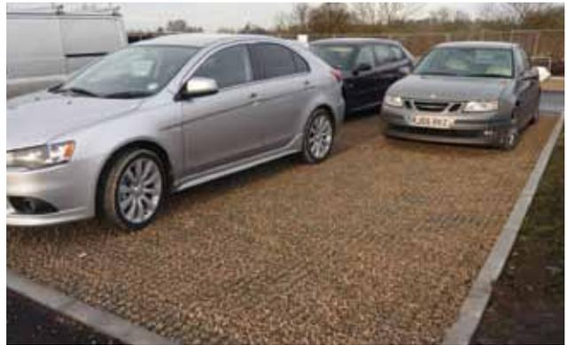
BODPAVE 40's open cell structure allows unrestricted healthy grass root growth and water infiltration and can be used as part of a Sustainable Urban Drainage Systems (SUDS). The paver grids also incorporate 25mm 'ground-spikes' on the base which fix through the adjacent paving grid's edge-loops to provide the entire structure with firm anchorage and structural integrity.
